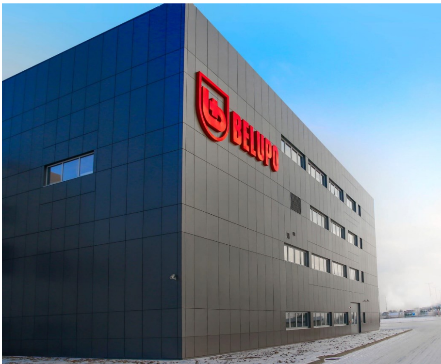
Figure 11. Headquarters of Belupo in Koprivnica, Croatia
